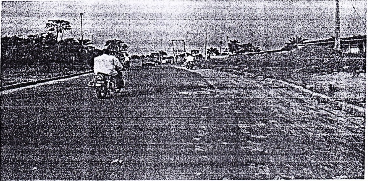
Plate 13: Asphalted road leading into Uta Ewa community.
